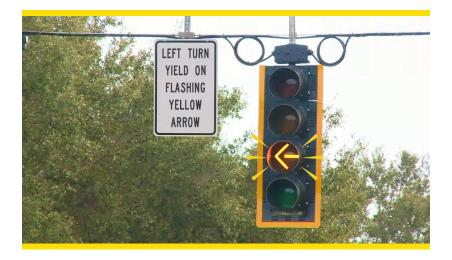
**WHAT:** Flashing yellow arrow signals are being installed at intersections throughout the state. The signal helps clarify to motorists to yield to oncoming traffic when turning left.
